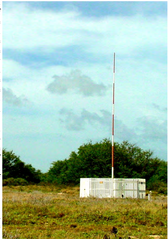
Figure 1.27. Fiberglass whip antenna at WWVH.
