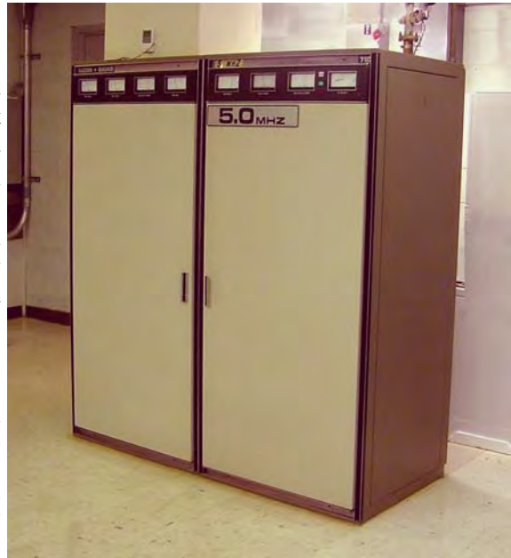
Figure 1.25. The 5 MHz transmitter at WWVH.
