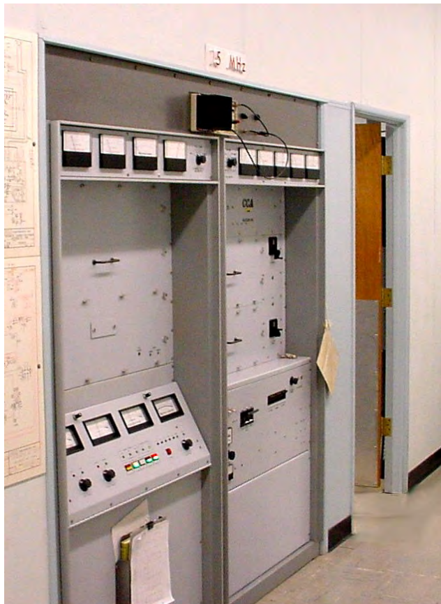
Figure 1.8. The 15 MHz transmitter at WWV.
