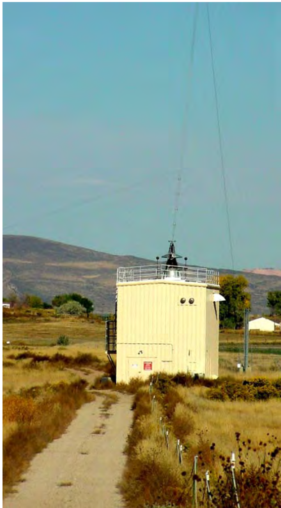
Figure 1.15. WWVB helix house.
