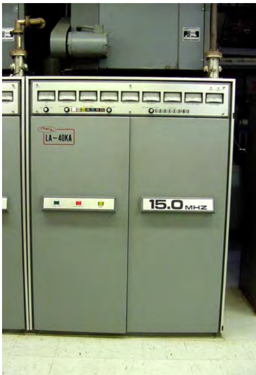
Figure 1.26. The 15 MHz standby transmitter at WWVH.
