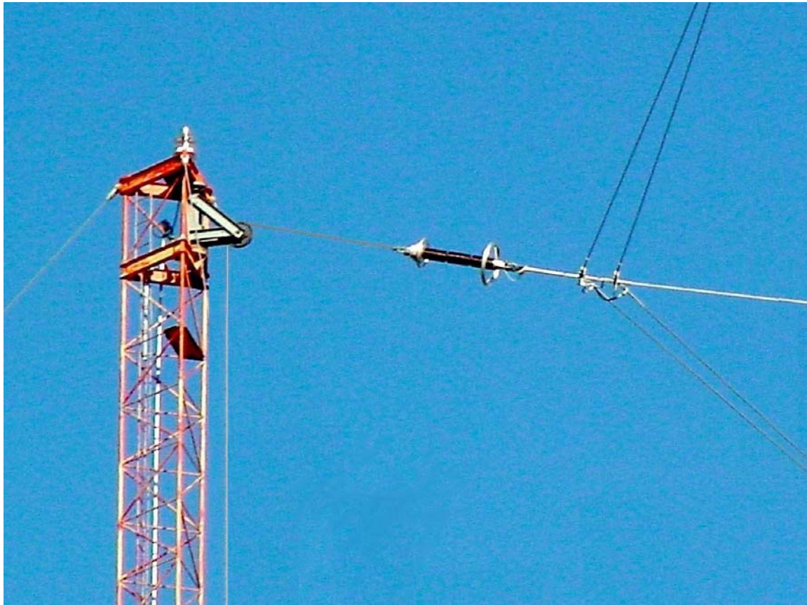
Figure 1.20. Antenna to tower connection detail.
