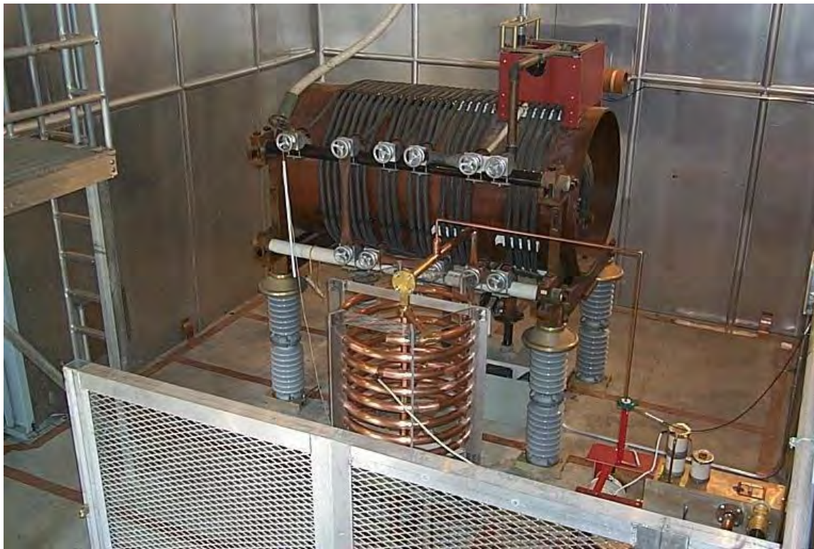
Figure 2.18. Interior view of helix house.
