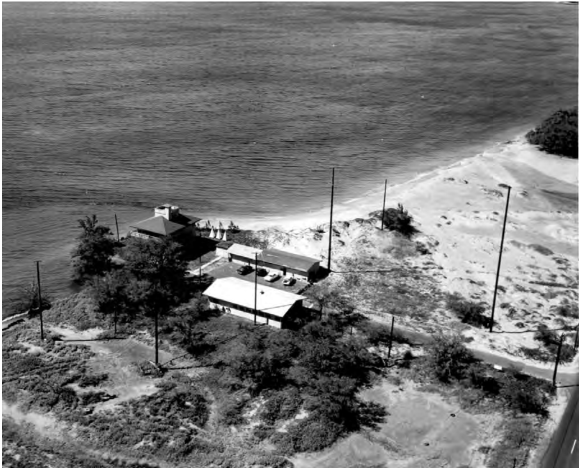
Figure 1.2. The original WVVH station site in Maui.
