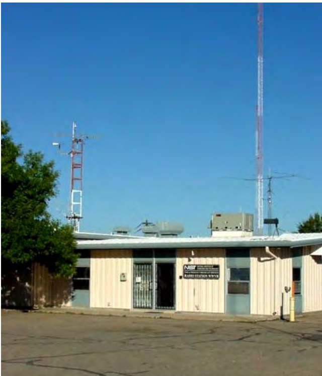
Figure 1.14. View of WWVB building.
