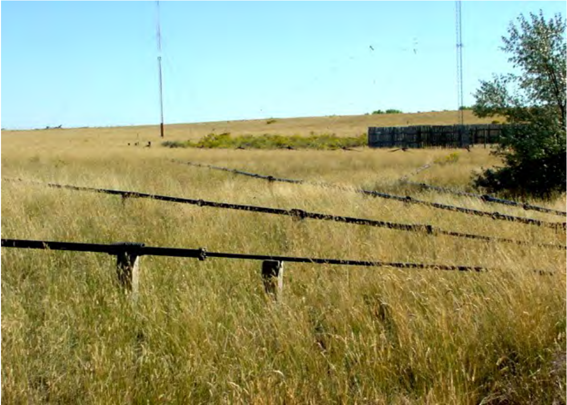
Figure 1.13. Transmitter to antenna transmission lines at WWV.
