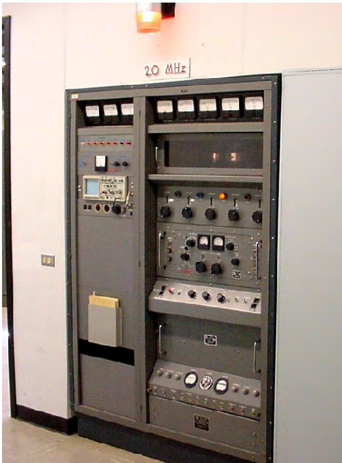
Figure 1.7. The 20 MHz transmitter at WWV.
