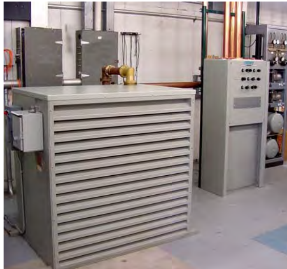
Figure 1.18. Dummy load and switch matrix..
